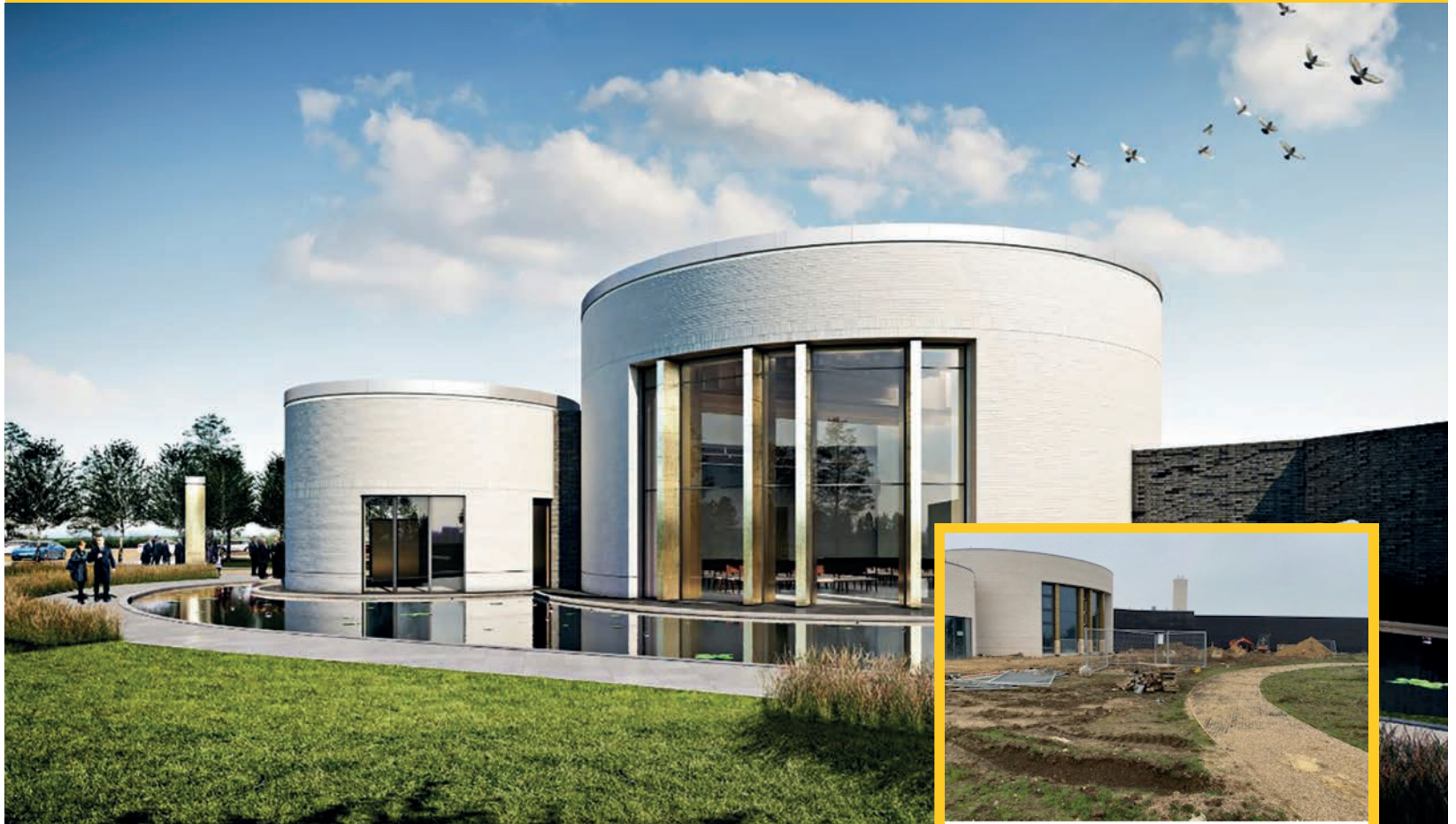
Development in Progress – March 2021
