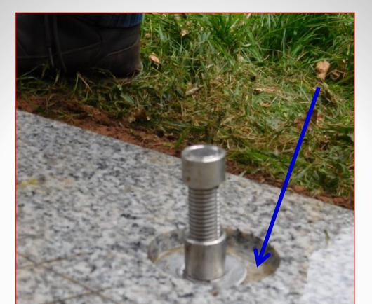
A memorial originally installed with a deep counter bore in the foundation may prevent a pin type anchor from engaging. (This generic photograph illustrates this point)
