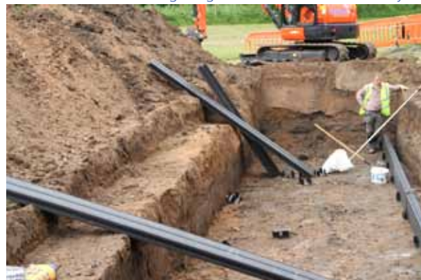
6. The serious business of getting it all in and level is under way.
