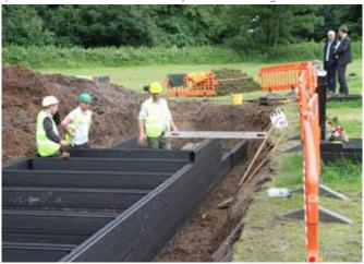
9. The internal grave spaces are backfilled in the same manner as with any grave space. The grave to the right of the picture is being left opened for the interment on Friday. A small amount of water can be seen on the inside right of the grave space.
