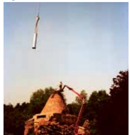
Lowering and guiding in the flue – with not much room for error – for the original single cremator installed within the kiln.
