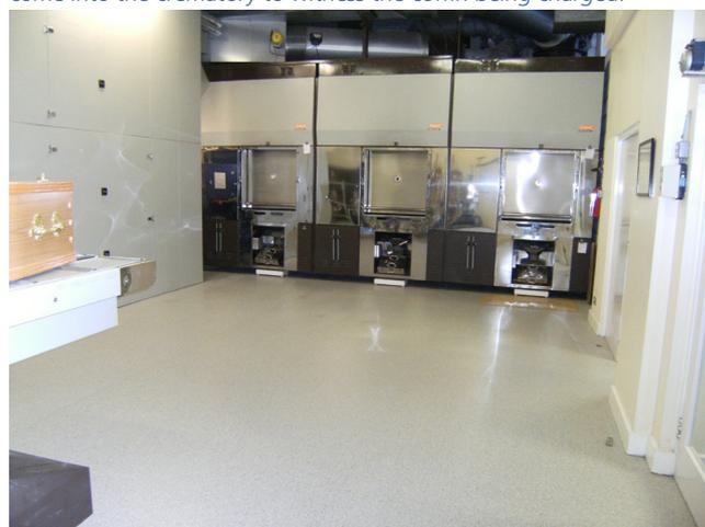
*Cremator No.2 and to the immediate left of it can be seen the end of the boiler which was slotted into the space vacated by the redundant No.1 cremator. To the very left is the edge of the screen surrounding the filter which stands in the space previously required to charge No.1 cremator.*
