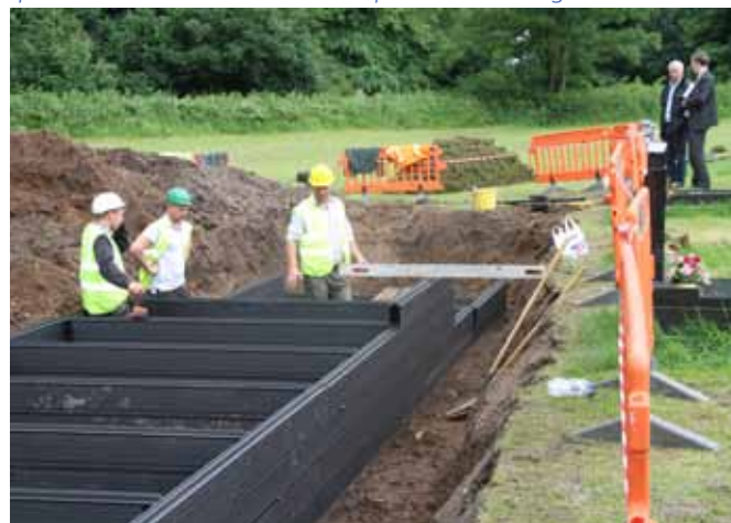
8. With the outer frame in and level the individual grave spaces are now being formed, 12 in total and the same dimensions as any other grave space 9' x 4'. As the units are built up so the backfilling continues.
